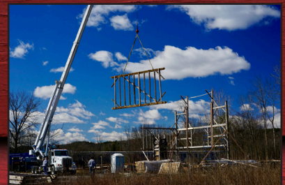
Placing a section
