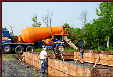
Pouring concrete for foundation
