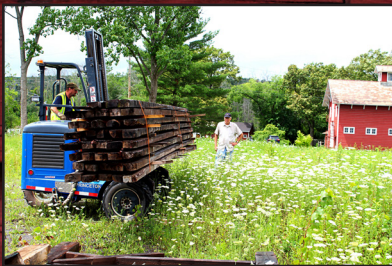
Delivery of original rafters
