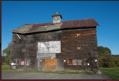
Barn before disassembly in 2017
