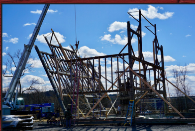
Bent 4 rising into place
