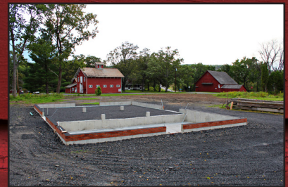
Completed foundation and brick ledge
